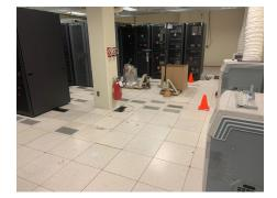
AFS was able to replace the entire access floor, clean the sub floor, and assisted in removing old unused utilities. After replacing the floor, AFS was able to optimize the position of dampers and directional air flow panels. By directing the cool air to the server load, the county is able to shut down an entire CRAC unit! Leading to thousands of dollars in annual energy savings!
