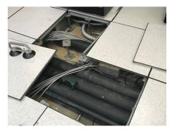
The 40 year old data center has seen several IT technology refreshes throughout its use, and the infrastructure supporting the IT function had reached the end of its serviceable life. A new CRAC unit installed in 2016 lead to new piping, conduit, and fiber runs that interfered with existing utilities creating a blockage in the underfloor plenum.
