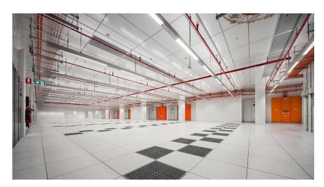
Tate Structural Ceiling Grid (SCG) is designed to support, overhead electrical buss duct, multilayer cable tray, lighting and fire suppression. Tate's SCG uses standard lay in acoustic ceiling tiles and lights, or can be configured to index with the access floor grid creating an alpha numeric layout for a data center.
